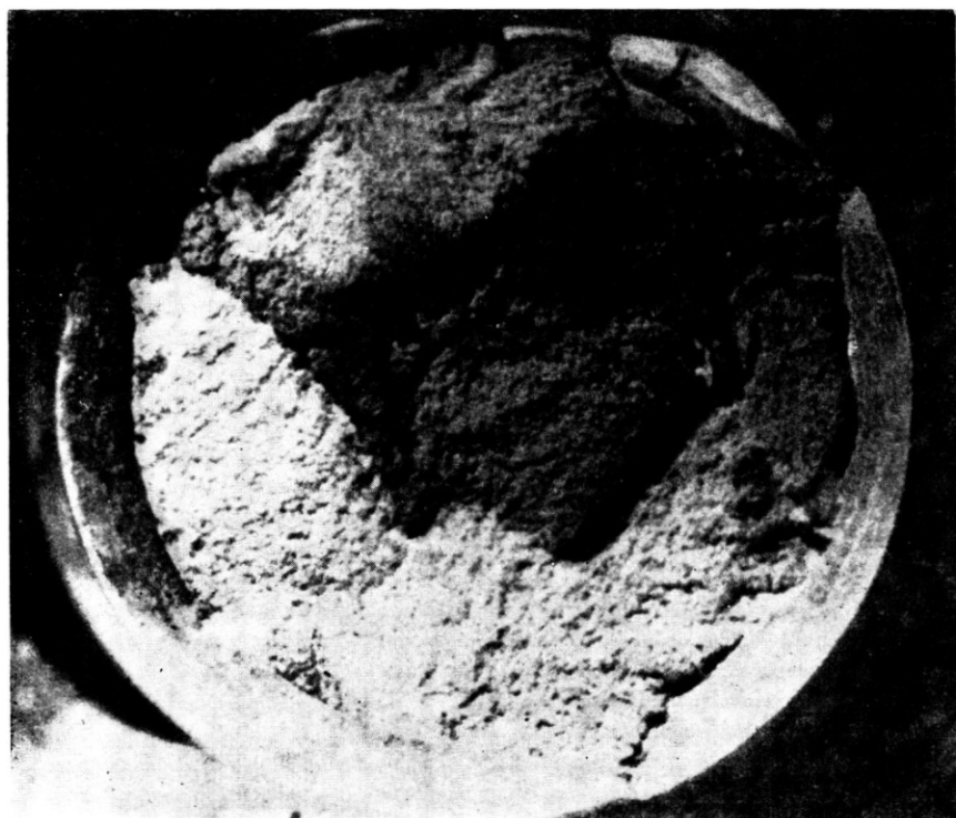
FIG. 1. Fracture appearance of a failed bolt.
